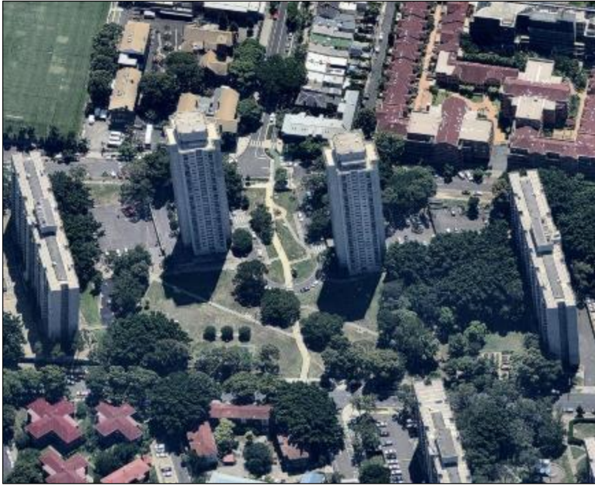
Figure 3-12 Tower development in the northern part of the Precinct. (Source: Nearmap)
