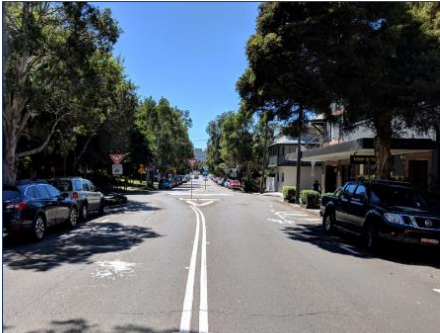
Figure 6-15 Henderson Road, Erskineville
