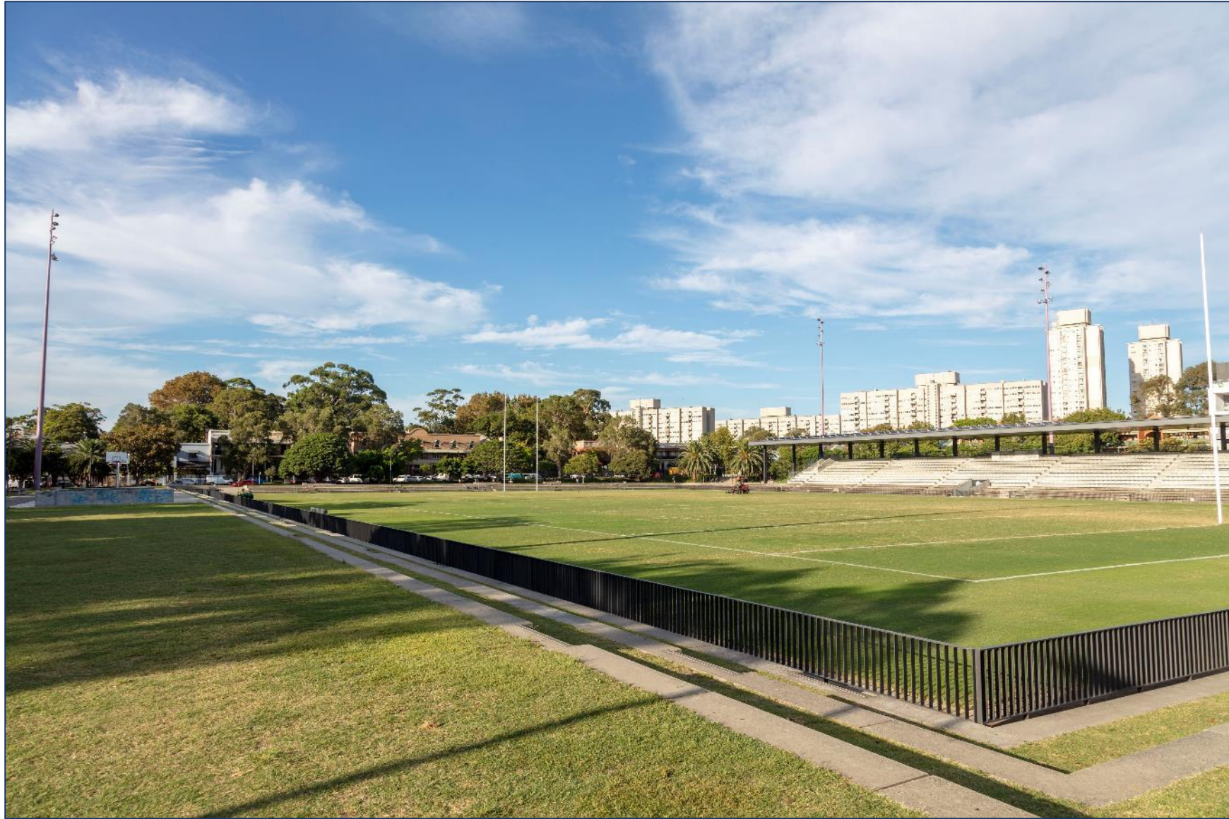
Figure 6-25 Viewpoint 7 – Redfern Oval, adjacent to north eastern edge of oval (current view) Source: Virtual Ideas
