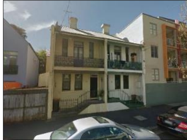
Figure 3-33 Remnant terraces, Cope Street.
